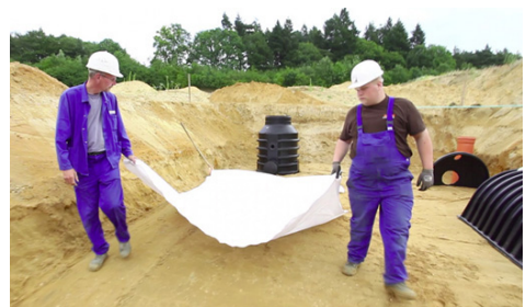
Image 7: Woven filter fabric on bottom area
