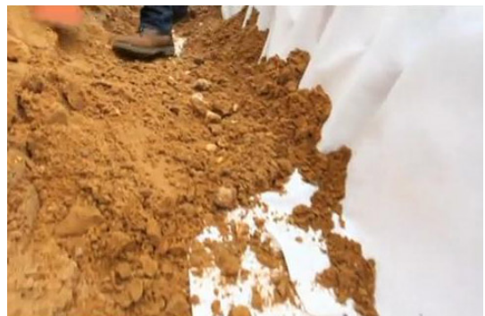
Image 11: Backfilling filter fabric for fixing
