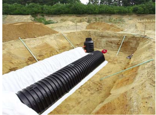
Image 10: Covering with filter fabric
