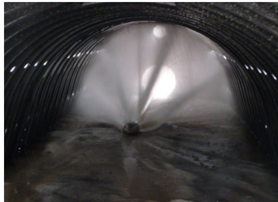
Image 4: Flushing nozzle with cleaning procedure
