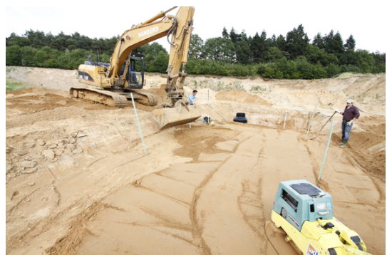
Image 13: Covering the tunnel elements
