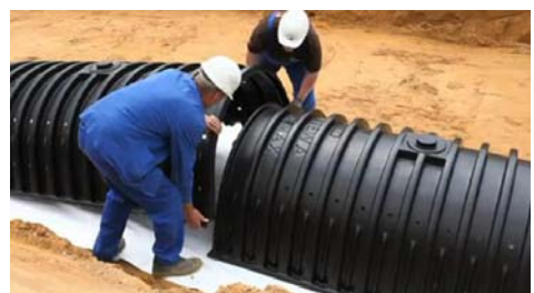
Image 9: Form lock fixing of two tunnels
