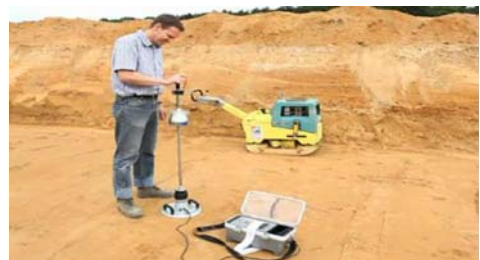
Image 6: dyn. Plate load test at ground level
